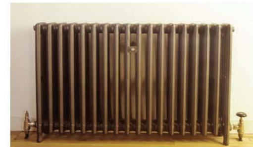
Figure 6.18 Baseboard heaters and radiators heat air by conduction with the air particles that come in contact with the metal surface. The hot air distributes the heat throughout the room by convection.
